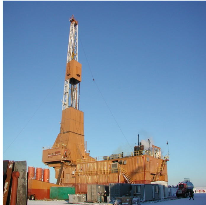
A large scale experiment on the Alaskan North Slope
